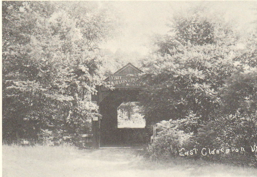
MILL RIVER (KINGSLEY) BRIDGE AT EAST CLARENDON Built by Timothy Horton
